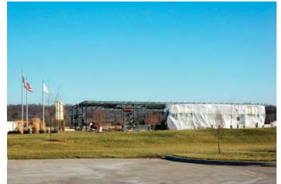
Construction is underway for a company new to Harrison
